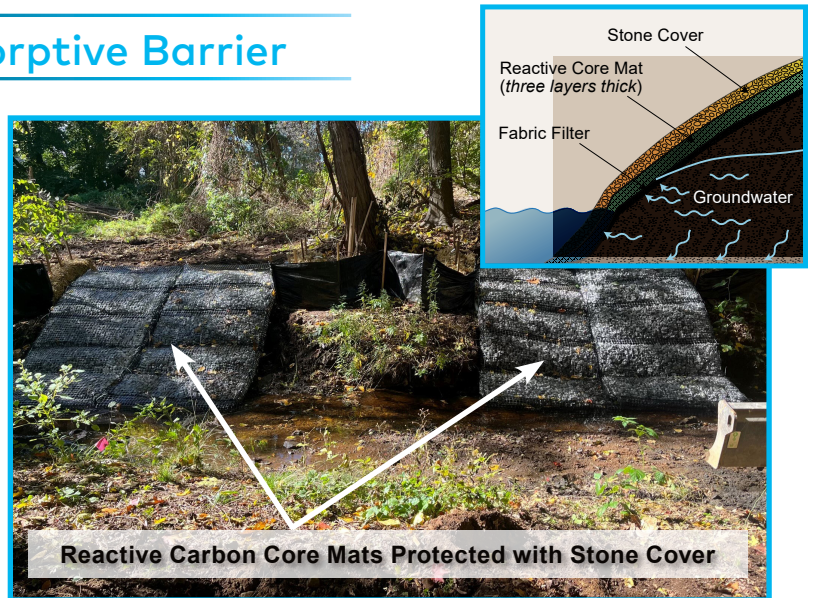
Figure 4 Reactive core mat installed at Stream A seeps
