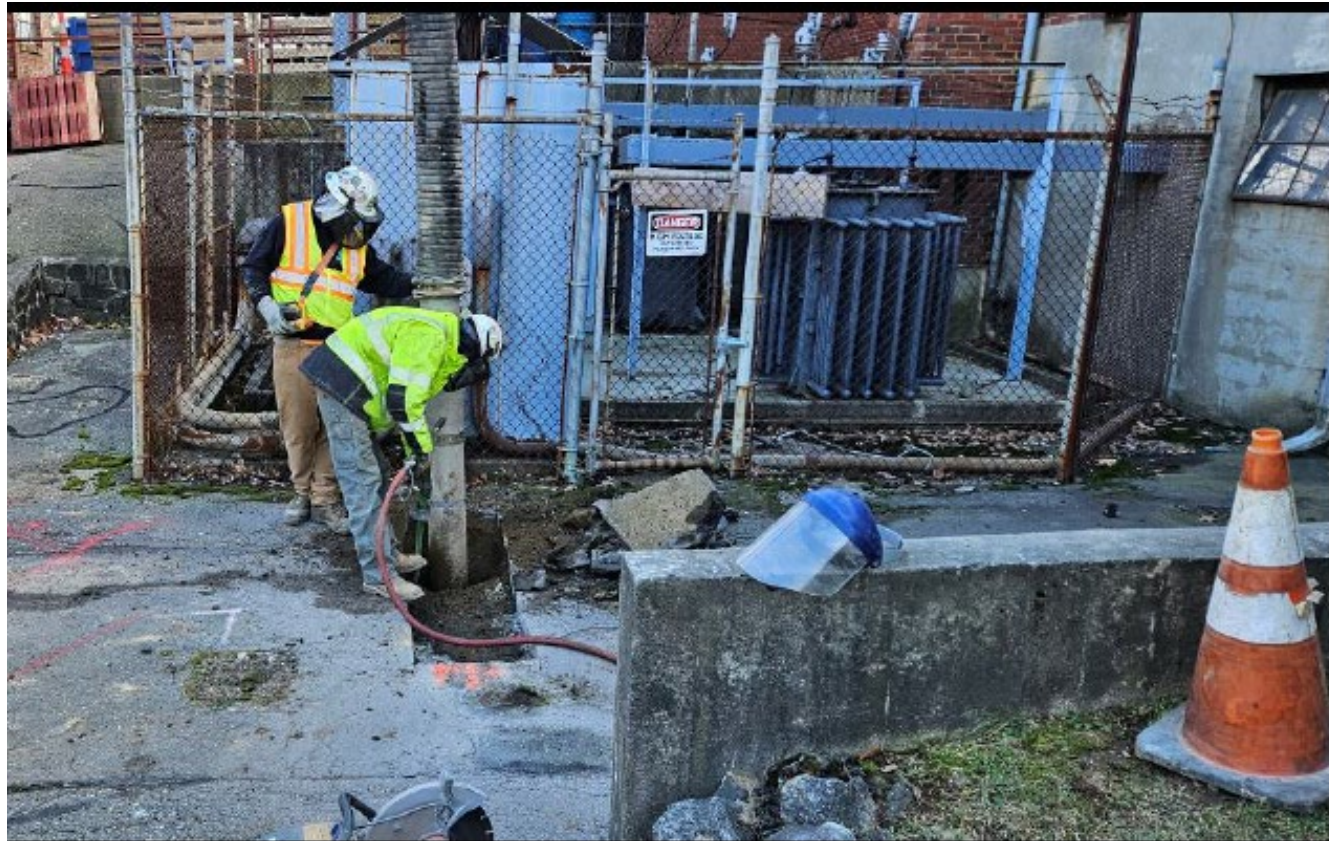
Material Removal by Vacuum
