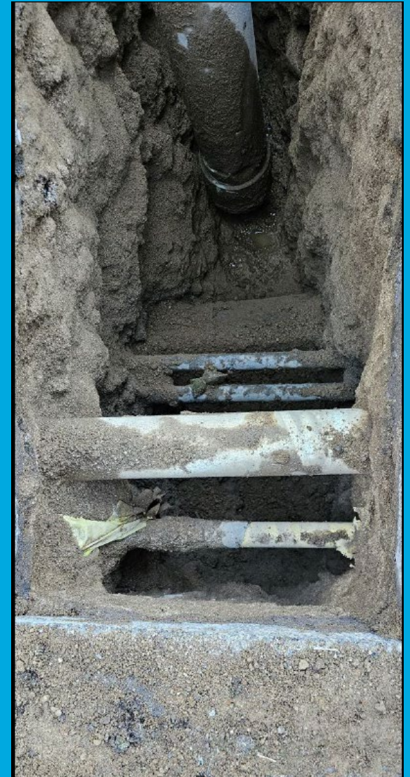
Uncovering buried utilities using “air knife” (prior to drilling)
