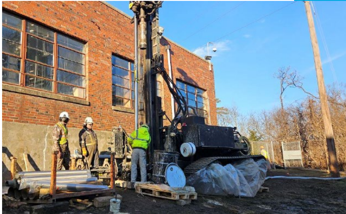
Heating well drilling and installation
