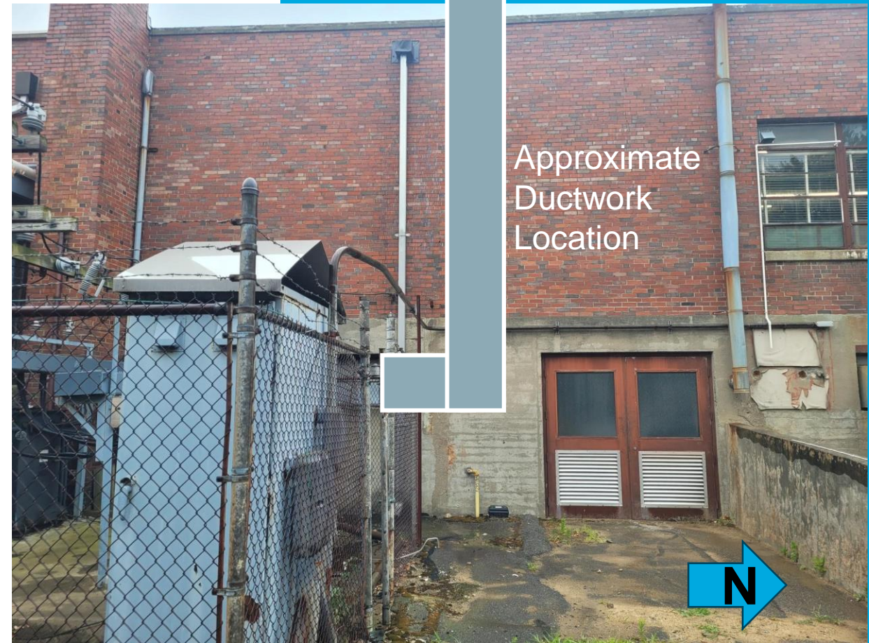
HVAC Equipment Upgrade Approach
