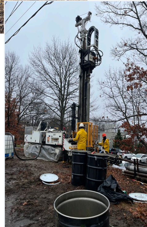
Recovery well drilling (Dec 2024)
