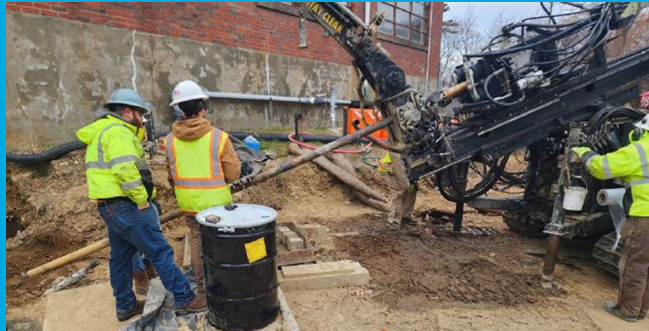
Angled drilling in Building 3 Area
