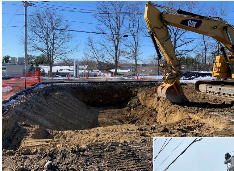
Soil excavation for SBGR (Jan 2025)
