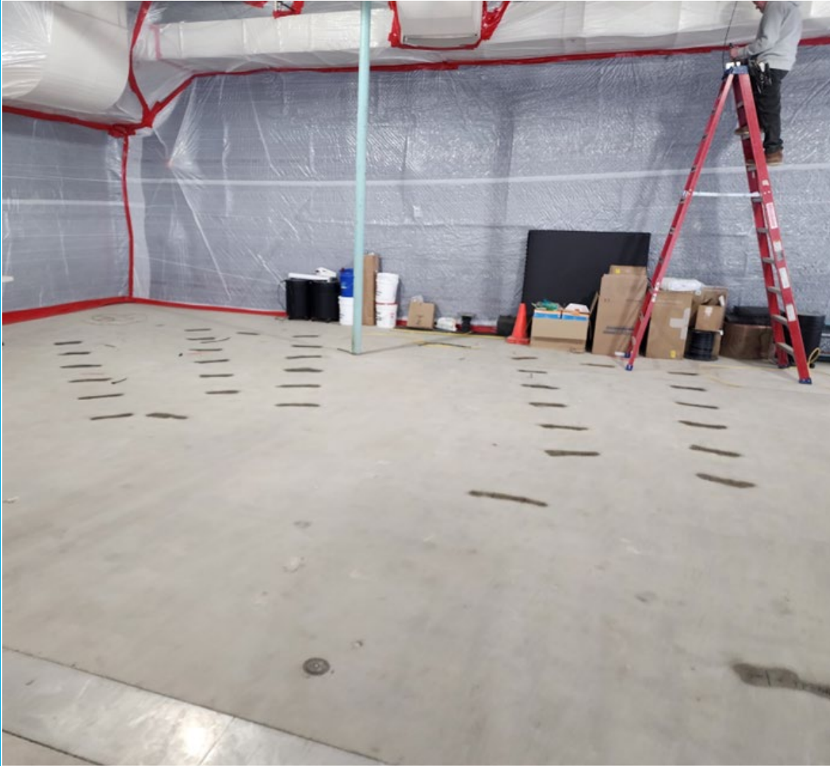
Sealing walls and conduits in the Building 3 stockroom (interior drilling area)
