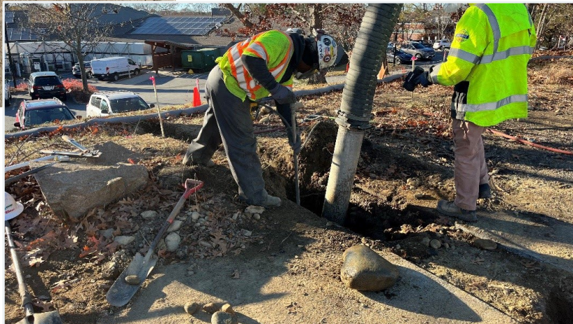
Soft digging to locate utilities (Nov 2024)
