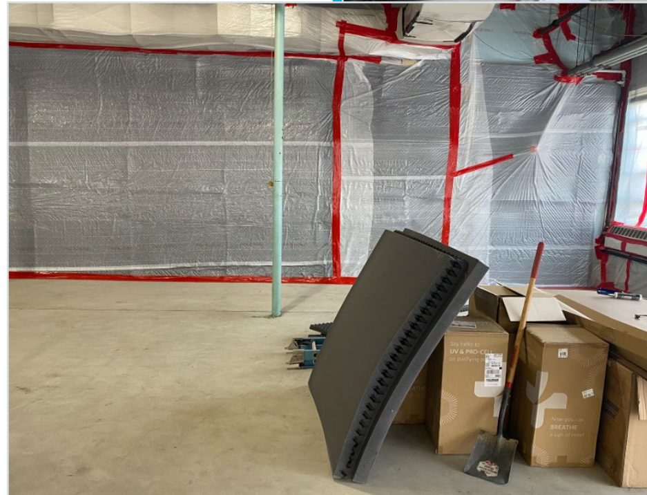
Sealing walls and conduits in the Building 3 stockroom (interior drilling area)
