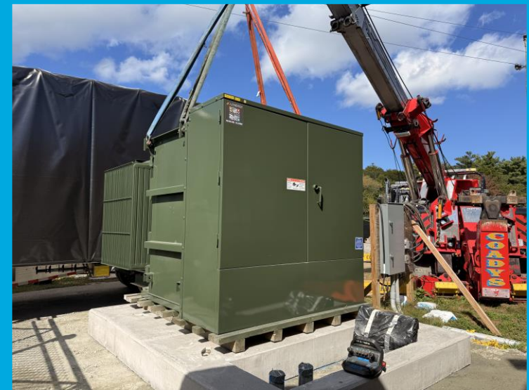
Electric transformer installation
