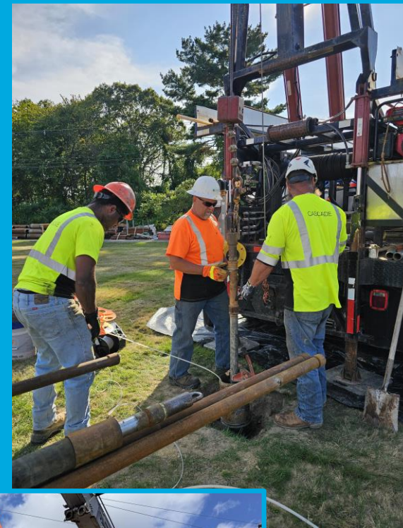
Bedrock packer installation
