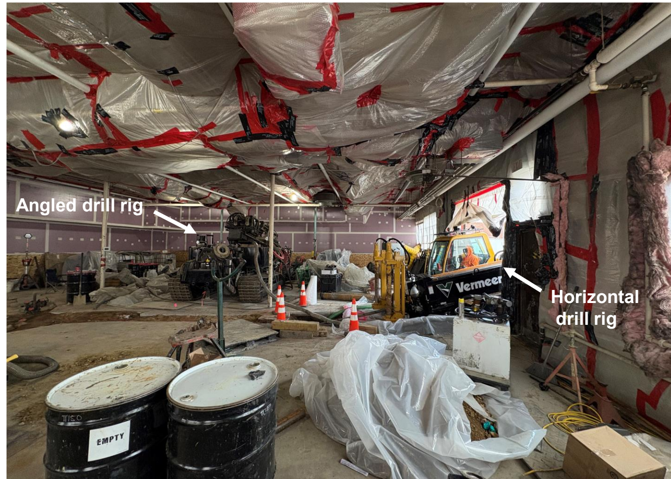
Stockroom drilling
