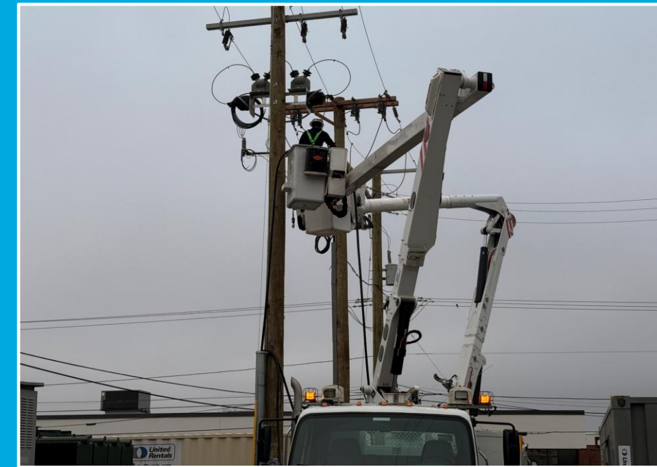
Power service installation
