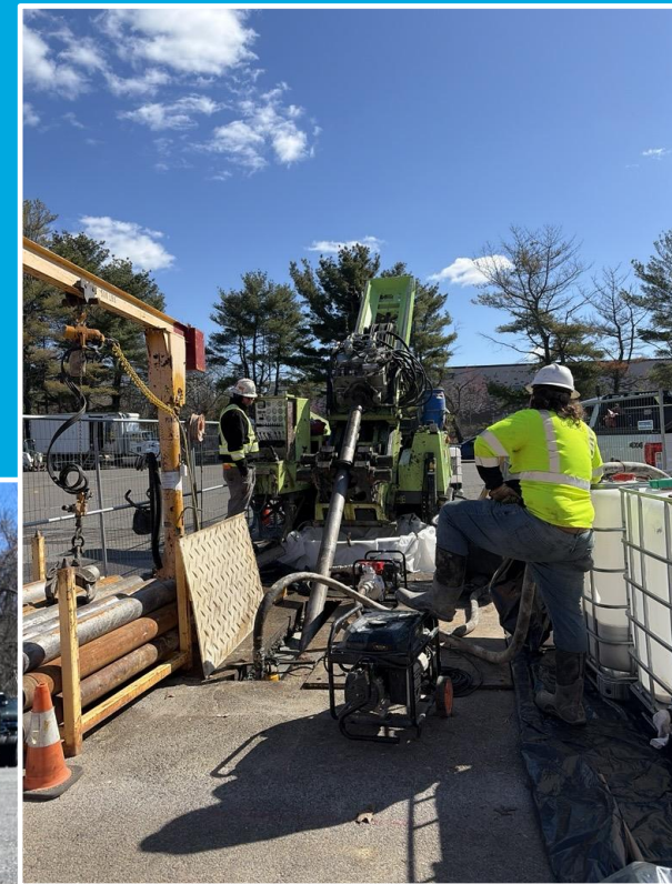
Angled well drilling near Building 5
