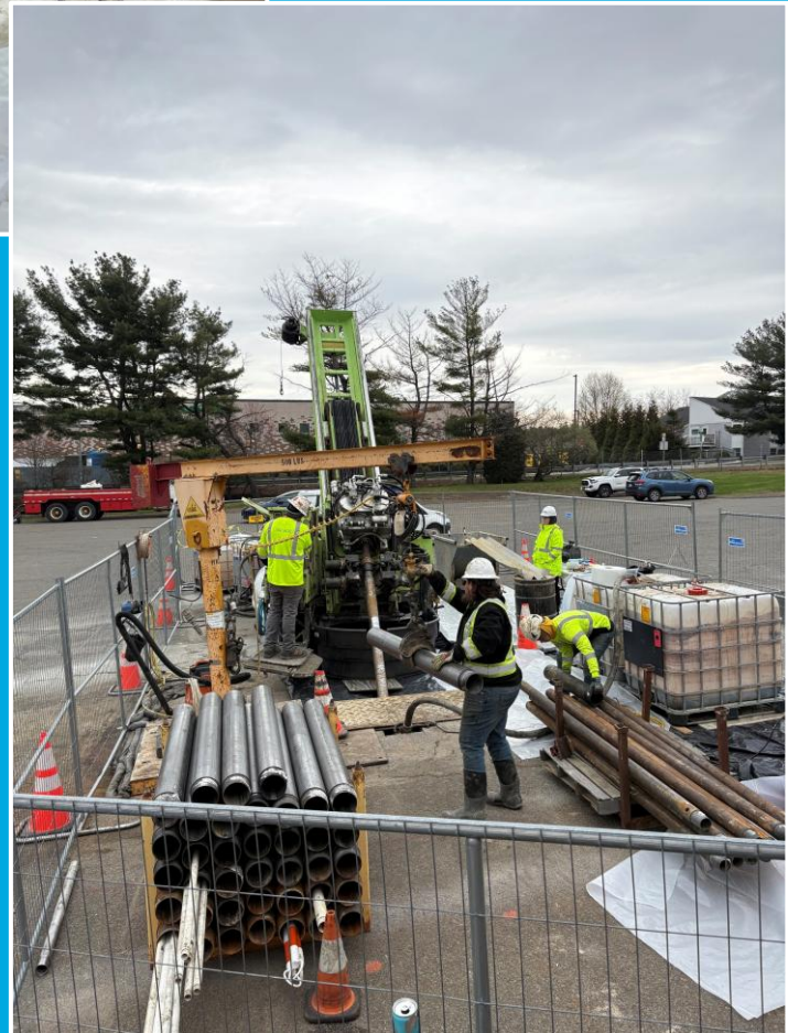
Angled well drilling
