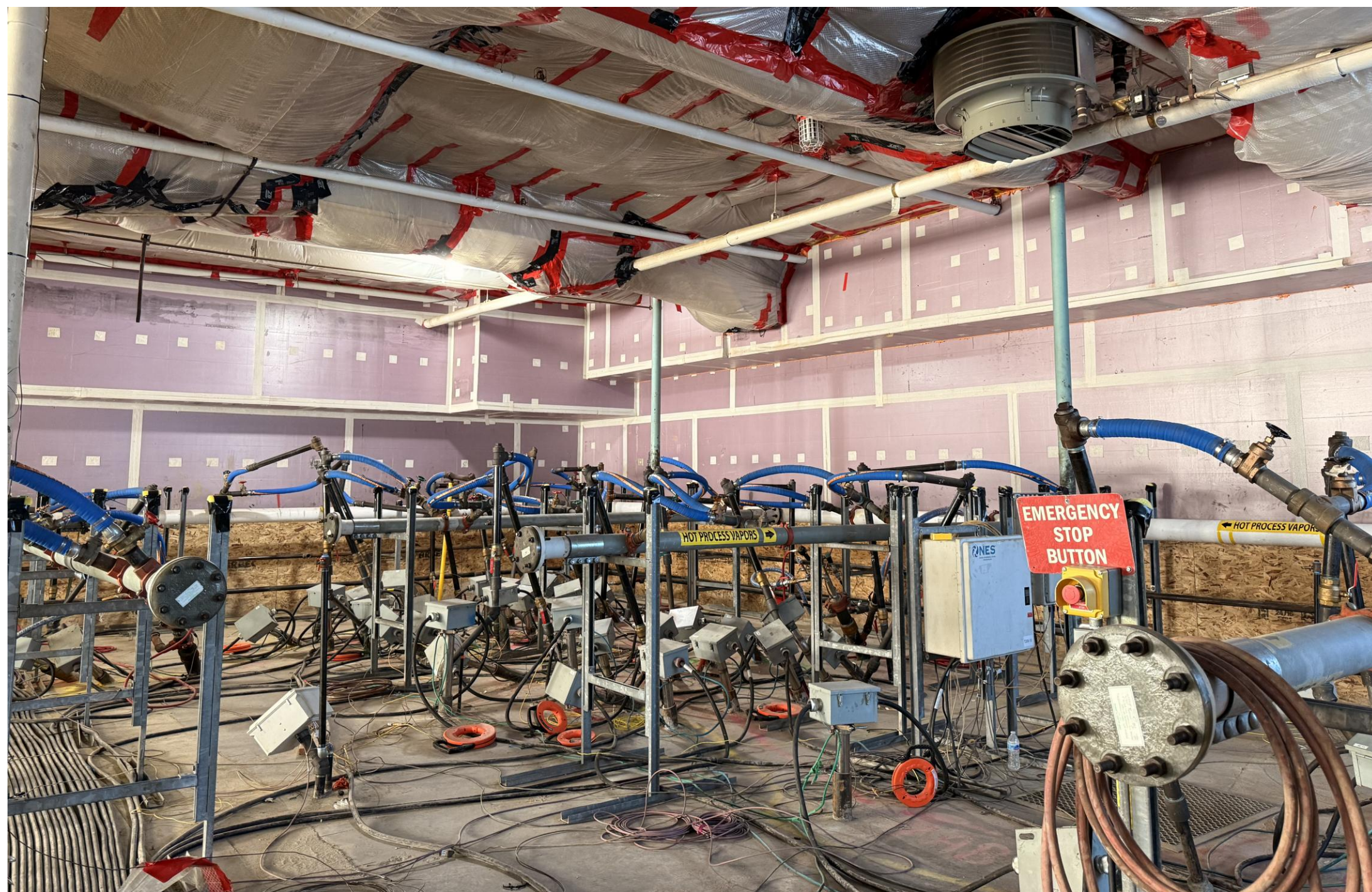
Completed Stockroom Installation
