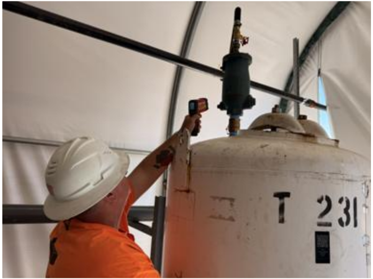
Treatment Process Monitoring
