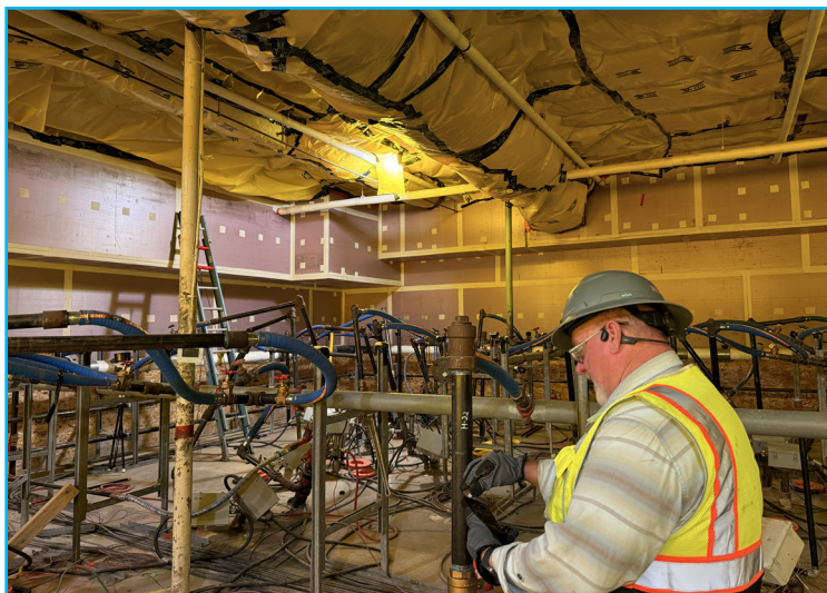
Figure 6. Drilling and installation of interior thermal wells
