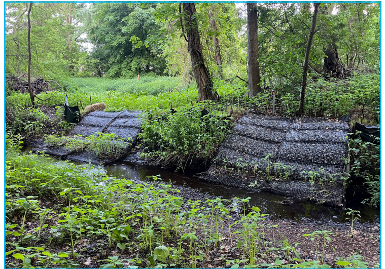
Figure 7. Stone covers reactive core mats along the stream
